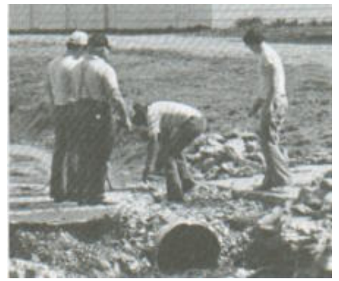
Bro. Wilson helping construct a new bridge on God's Acres.
